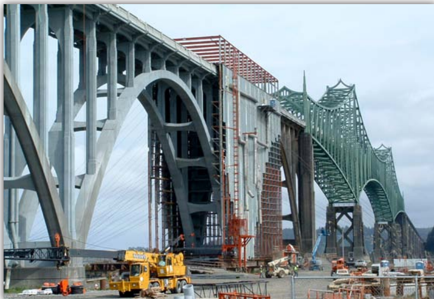
Left: US 101 McCullough Bridge (North Bend) – Hamilton has a tremendous amount of experience with cathodic protection systems on the Oregon coast. Here, the work bridge provides a safe work environment and contains dust during cathodic protection work. Above: Siuslaw River Bridge – Art deco on the outside – high tech on the inside.
